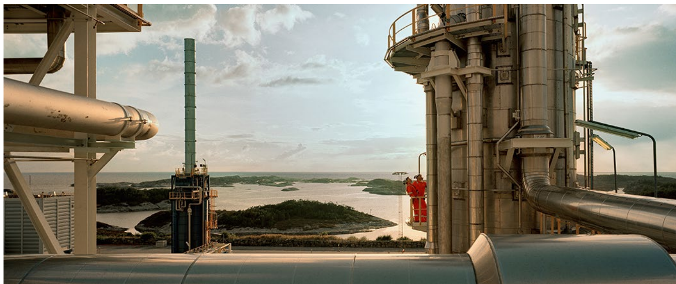
Kollsnes gas processing plant at Øygarden, Norway.
